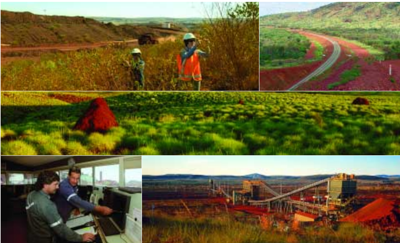
The Southern Spur Rail Project has set a new industry benchmark for the construction of a low-impact railway.
